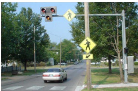
Pedestrian activated warning signals with signage at a midblock crosswalk
