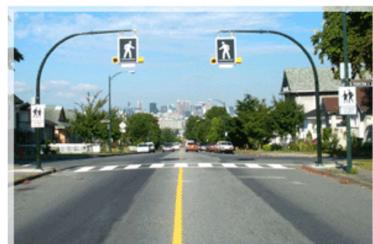
Warning signals with signage can alert drivers to crossing pedestrians at an otherwise unsignalized intersection
